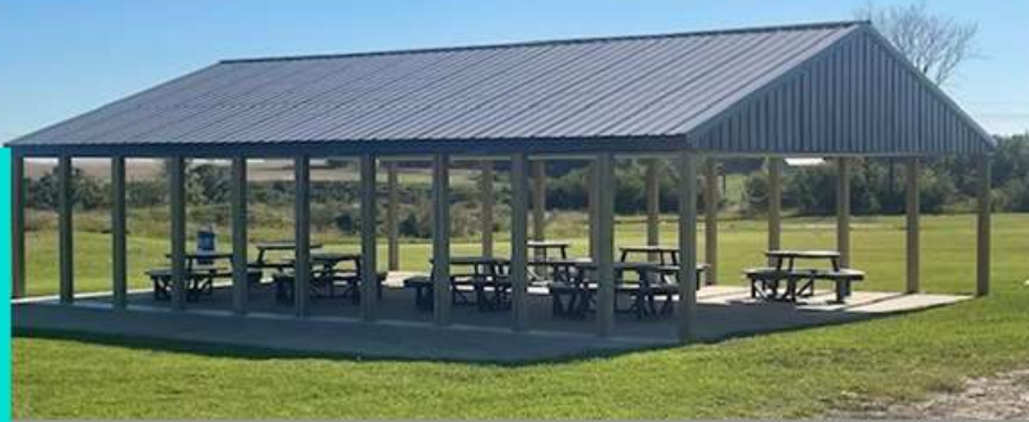
New outdoor classroom, photo: Bry Sabry
